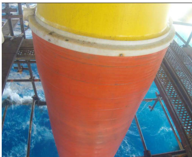
Figure 18—Completed Helicoid Epoxy Sleeve System
