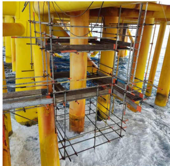
Figure 14—Scaffolding Erection
