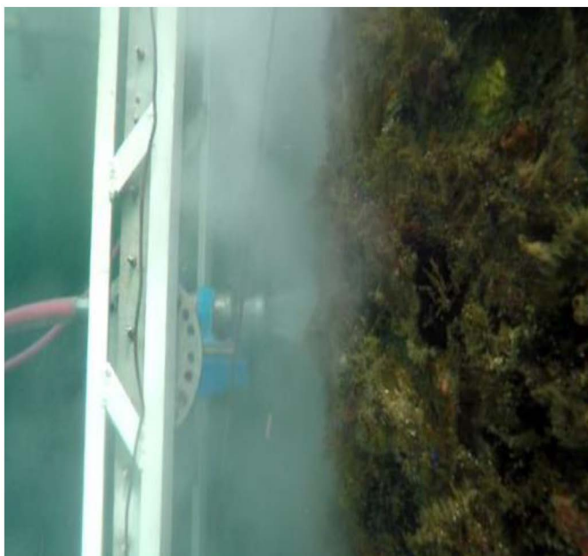
Figure 15—Surface Preparation Underwater
