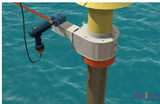
Figure 9—Insertion of Carbon Fiber Reinforced Strip
