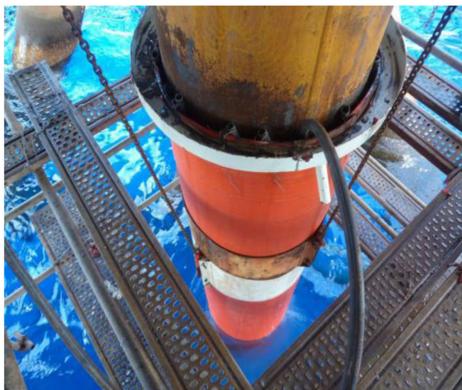
Figure 17—Injection of Epoxy Grouting
