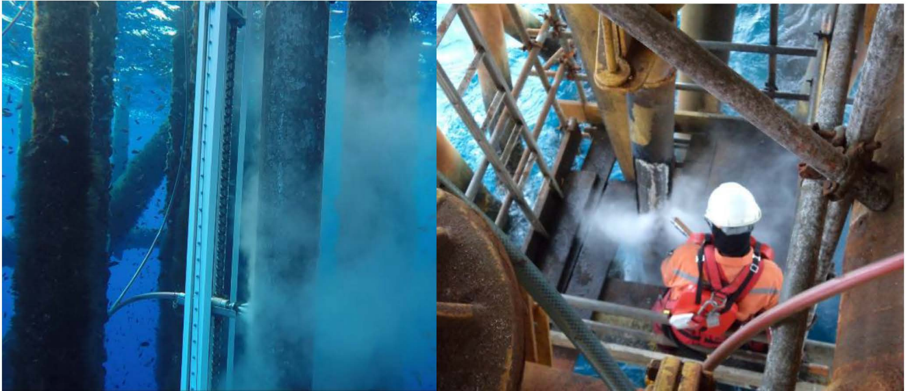
Figure 7—Riser Surface Preparation by Hydro Blasting for Underwater and Above water
