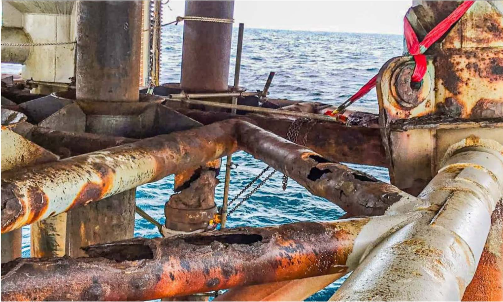
Figure 2—Perforated and Parted Conductor Casing
