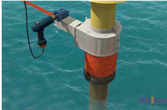
Figure 10—Fixing of Polyamide End Cap
