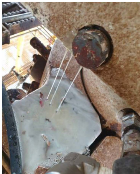
Figure 16(a)—Unknown plug leaked when performing pressure test diagnostic on well W3.
