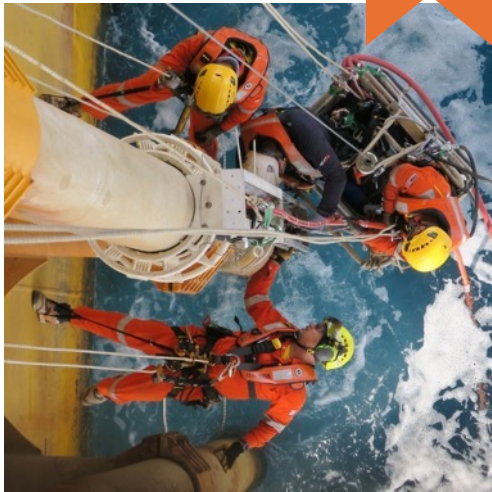
Blasting Frame Installation
