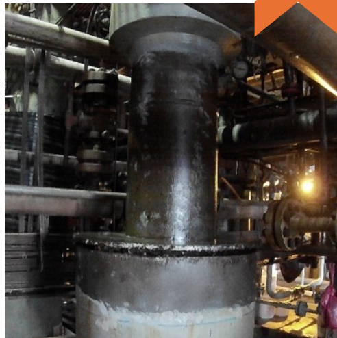
Condition after surface preparation
