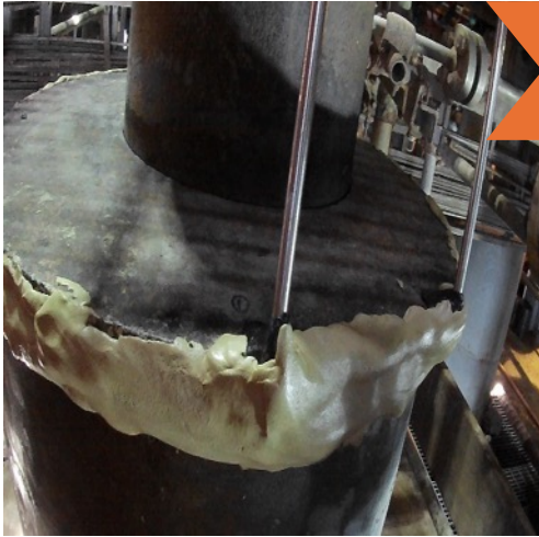
Vent Line Installation
