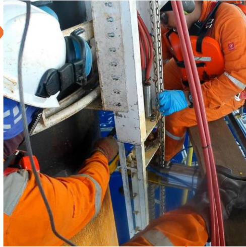
Helicoid RSS Installation
