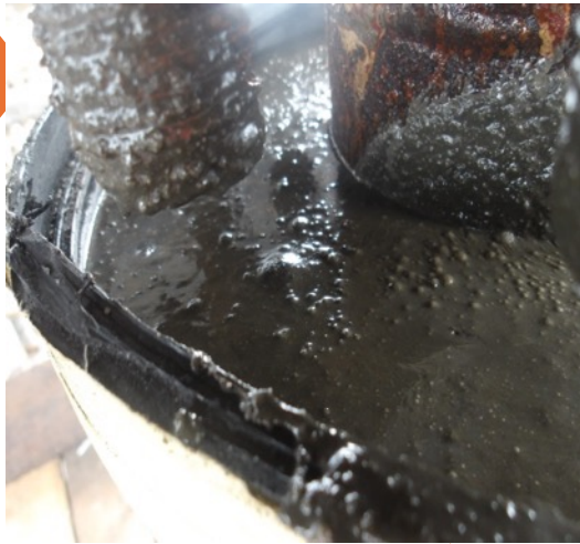
Epoxy Grouting
