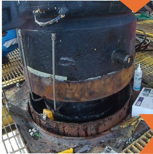
Leak Containment & Tubing Installation
