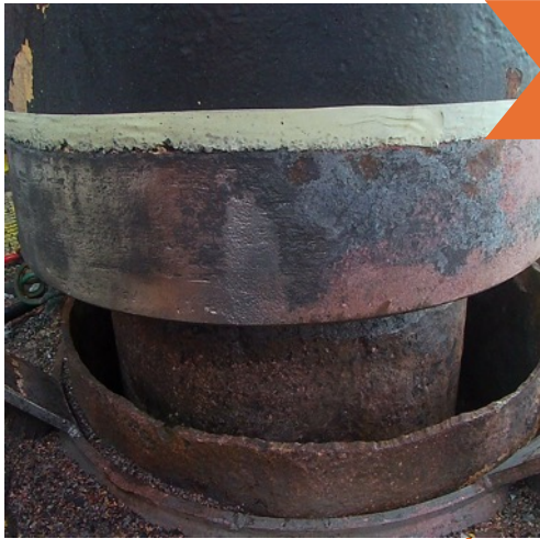
Existing Cement Removal
