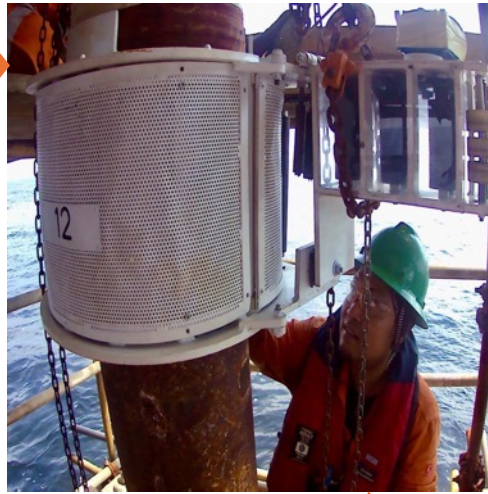
Winding Cage Installation
