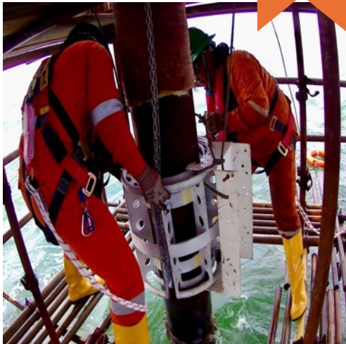
Pipe Bracket Installation
